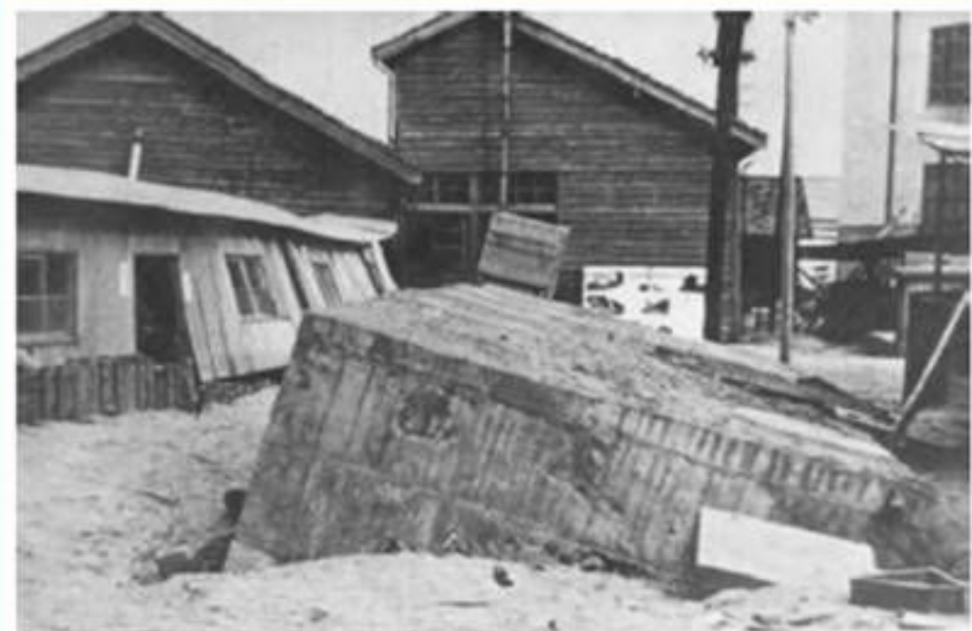
Figure 4. Floating of buried tank in liquefied ground, caused by the 1964 Niigata earthquake (photo: Kawasumi 1968).
