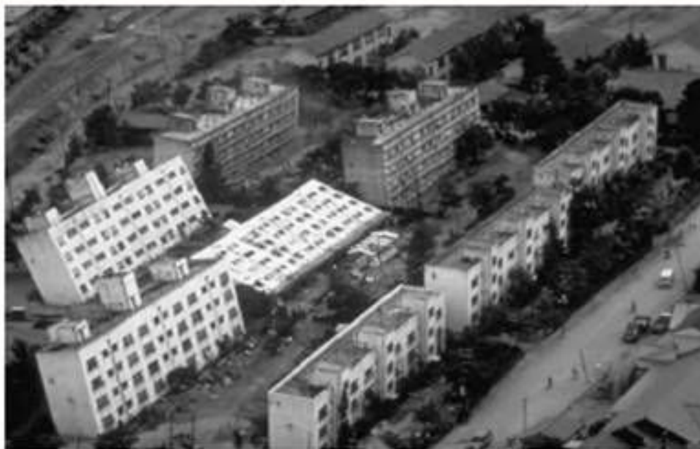
Figure 3. Tilting of apartment buildings caused by the 1964 Niigata earthquake (photo: National Information Service for Earthquake Engineering, EERC, University of California, Berkeley).
